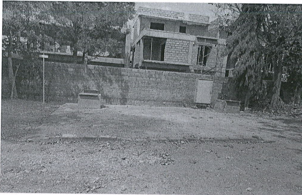
Bore well sump
